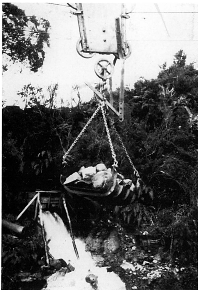
A stoning tray being used to remove excess rock rubble from a operation, West Coast, South Island, New Zealand (Department of Conservation collection, Westland).
