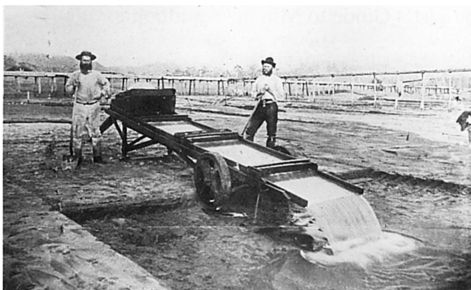
Fig. 1: A portable gold table being used for black sanding at Charlestown, West Coast, South Island, New Zealand. Note the wooden flumes in the background (Department of Conservation collection, Westland).
